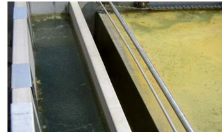
↑ Without chemical flocculation, the F.O.G floating on the surface
