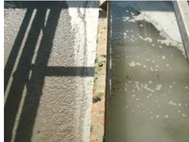
← Following the chemical flocculation, scum and floc-sludge floating to the surface and scrapped by skimmer system
